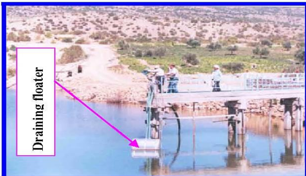
Attachment of the draining floater to a fixing system fixed to a footbridge
