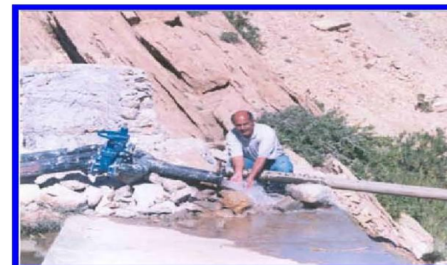
Water is flowing from a tap after priming the draining floater system
